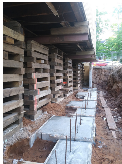
Re-building the west wall
